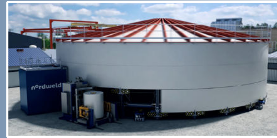
8. Assemble the 3rd course and so on until the tank reaches the final height.
