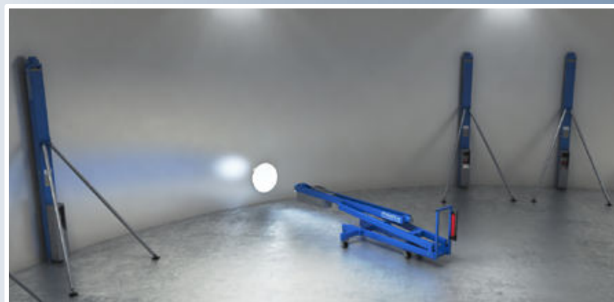
10. Remove the equipment and place the tank at the bottom and dismantle the Lift Jacks.
