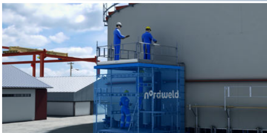
9. All NDT can be performed at ground level from one location.
