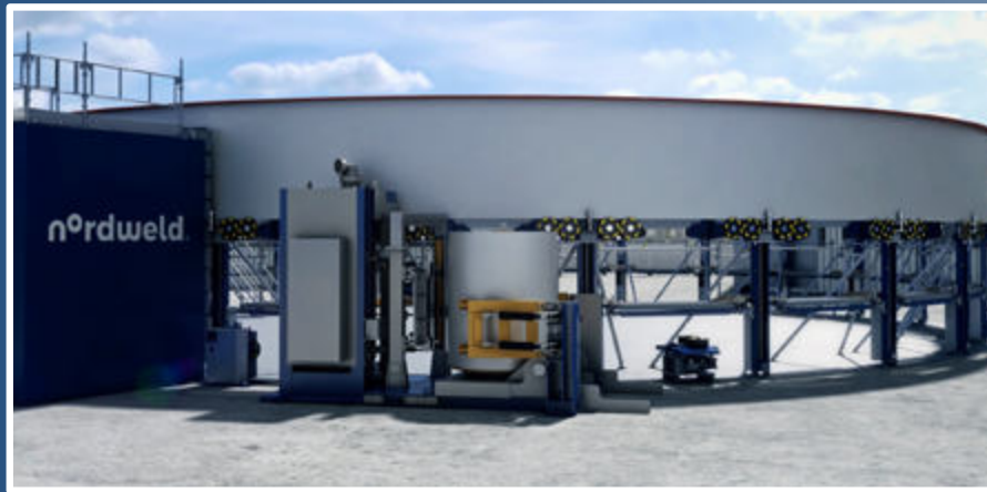
5. Lift the 1st course including the top ring.
