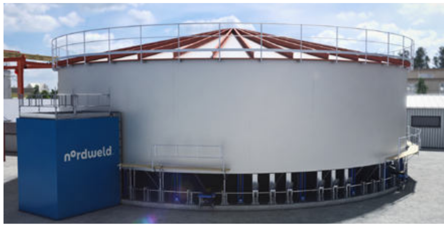
7. Lift the entire tank.
